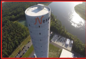
Goose Creek Plant, South Carolina, USA Land High Voltage Cables Update for Submarine High Voltage (2020)
